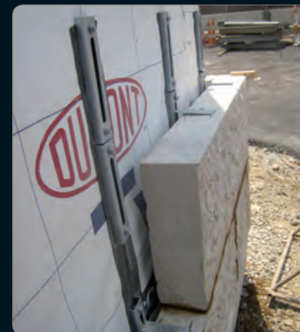
Full Veneer - Mortar setting with securing ties
