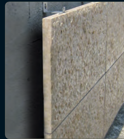
Full Veneer - Mechanical anchor fixings
