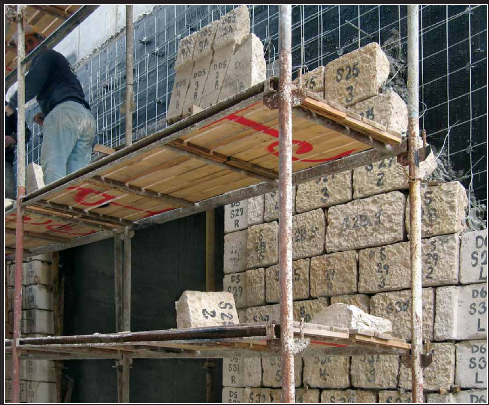
Mamilla, Alrov Quarter, Jerusalem, Israel. Renovation of an old building in Jerusalem. Each stone was assigned a number before dismantling the building and was reinstalled on the new building according to the numbers.
